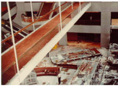
Locations of the second and fourth story walkways which collapsed; The third story walkway was offset by several m.
