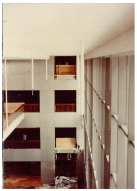
Locations of the second and fourth story walkways which collapsed; The third story walkway was offset by several m.
